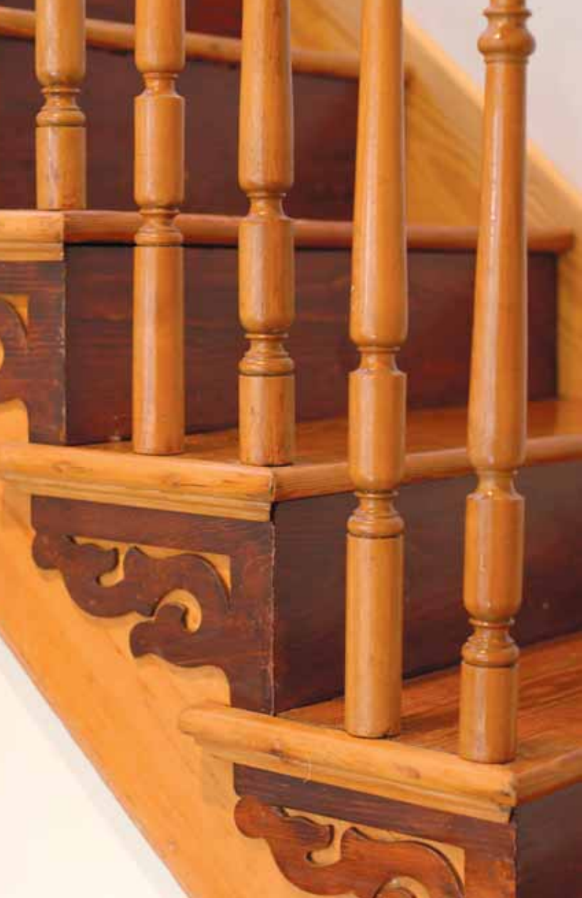
The spindles, trim and risers of these historic stairs were all taken apart, cleaned and put back together.
